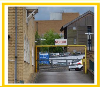
Height Restriction Barrier and Swing Gate combination is a highly effective deterrent for both controlling access to the carpark, as well as limiting the type of vehicles entering the area. The swing gate can be locked to prevent all access to the car park when required and opened to allow low vehicles access. This is a very popular option with country parks, schools, and public carparks with limited opening hours
