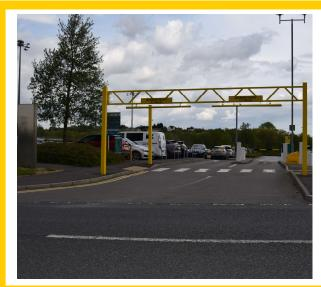
Heavy Duty Height Restriction barrier manufactured from heavy duty steel box section to offer additional strength and protection. This is an effective method of preventing unauthorised access to any high sided vehicles such as truck and caravans. Manufactured from heavy duty galvanised steel and painted finish to provide a durable and effective height barrier.
